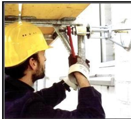
Fixing the scaffold to the building (construction, superstructure)
