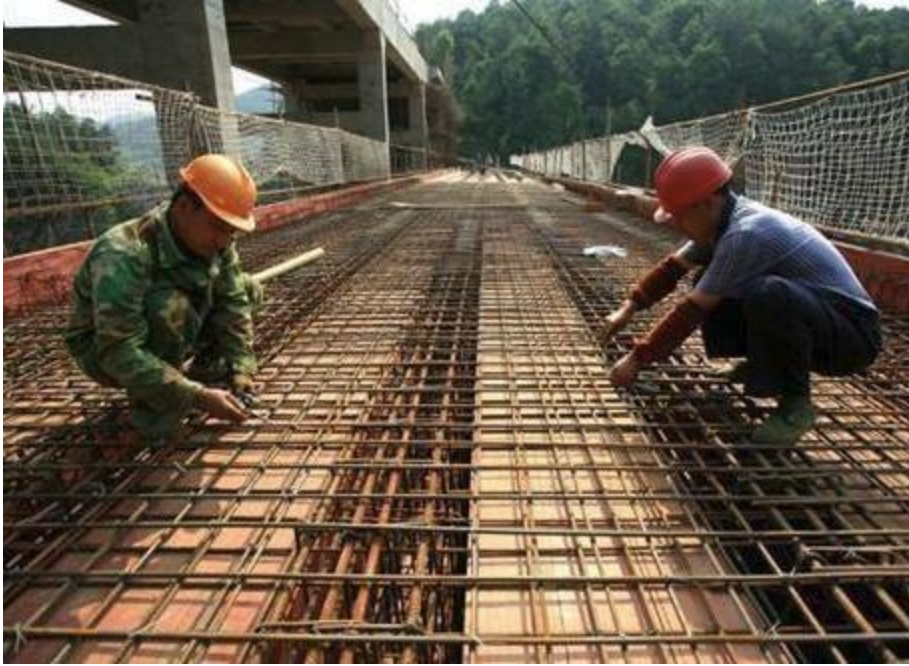
Installation of reinforcement on the site
