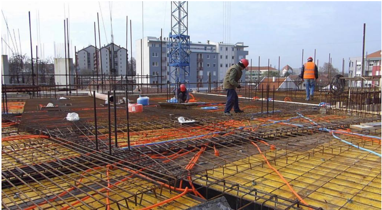
Installation of reinforcement on the site
